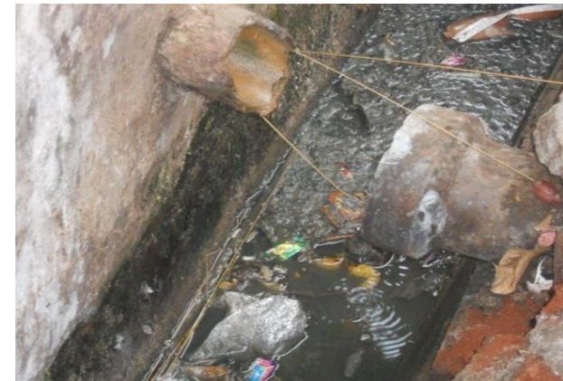
Toilets directly connected to drains
