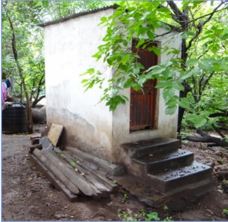
Septic tanks are below the toilets and don't have access covers
