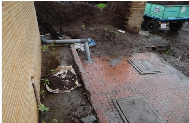
Oversized septic tanks
