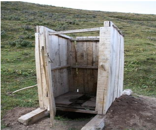
Single pit toilets
