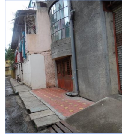
Septic tanks located near drains and sealed from the top
