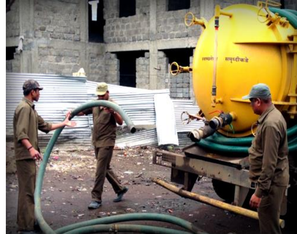
Unsafe handling of septage
