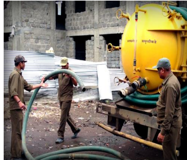
Unsafe handling of septage
