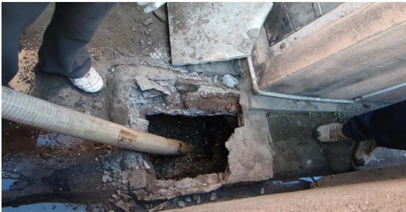
Emptying when the tank is full
