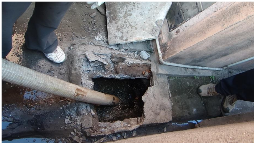
Emptying when the tank is full
