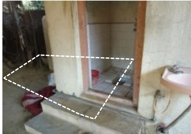
Inaccessible septic tanks with sealed tops
