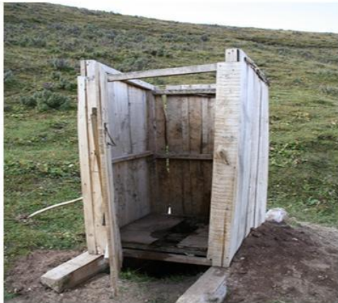
Single pit toilets
