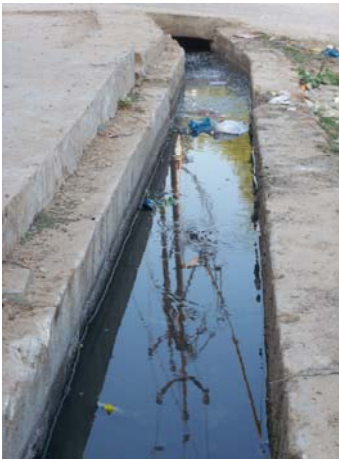
Sewerage – Open Drain (Picture : Patan)
