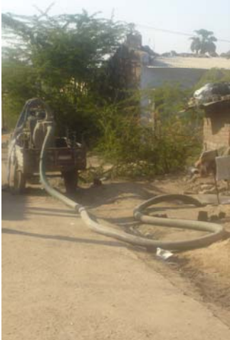
Drainage Cleaning (Picture: Kalol)
