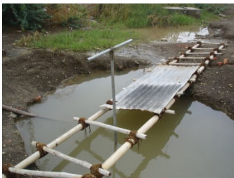
Leaking Valve, Morbi
