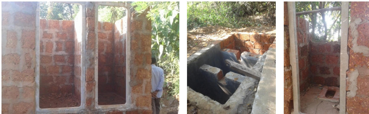
Photograph 6: Construction of individual household level toilets under SMMU
