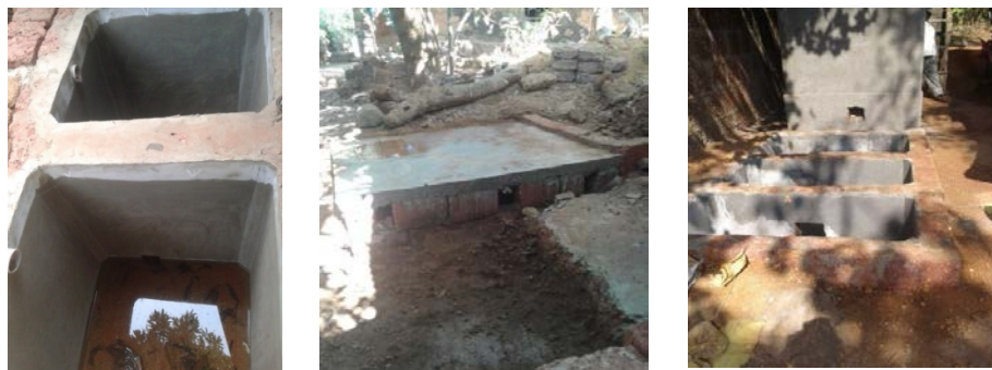
Photograph 7: Construction of septic tanks under SMMU
