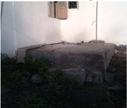
In many toilets, septic tanks located behind the complex
