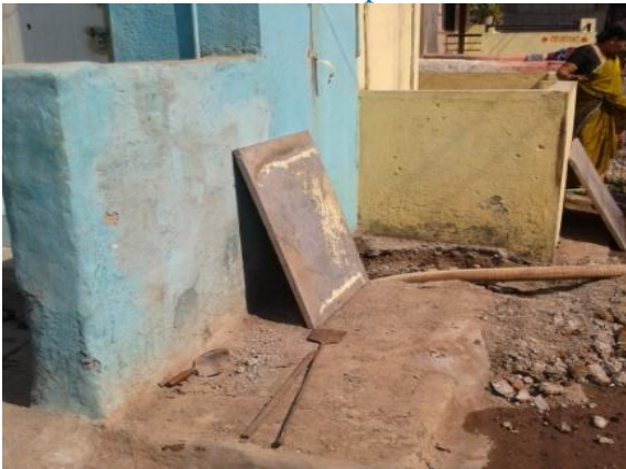
Inaccessible septic tanks with sealed tops
