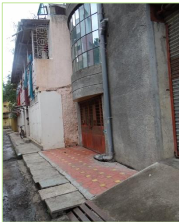
Septic tanks often empty into drains
