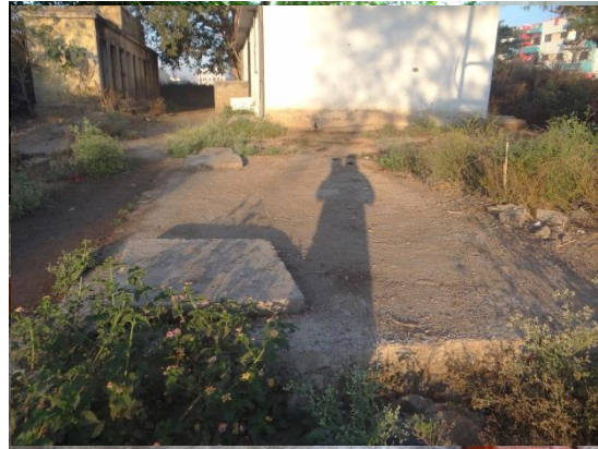
Some of the newer toilets have 2-3 chambered septic tanks with access covers
