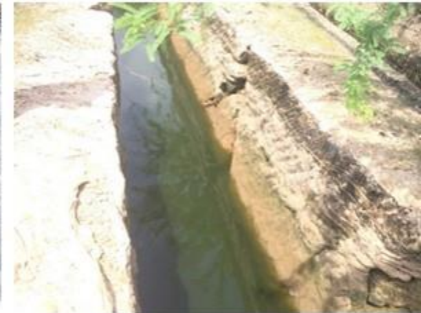
Canal linking the catchments
