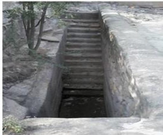
Water conservation and ground water recharge
