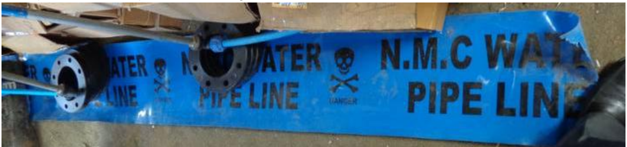
Hazard Plastic Tape laid by NMC over its water supply pipes to avoid accidental damage during excavation works
