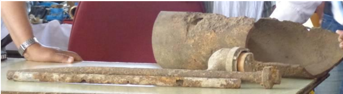
Corroded pipes replaced in the pilot zone of NMC
