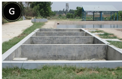
Sludge Drying Bed
