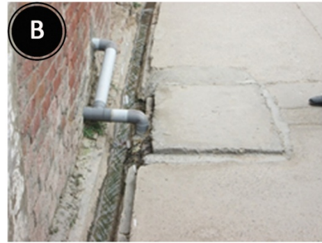
Intersection Chamber/ Septic Tank
