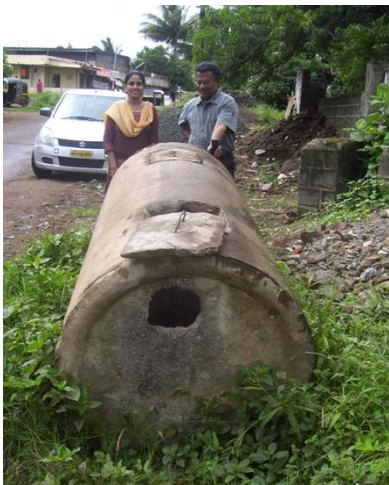
Figure 5 Local Innovation- Readymade Septic Tanks of RCC and Plastic used in Maharashtra & Jharkhand
