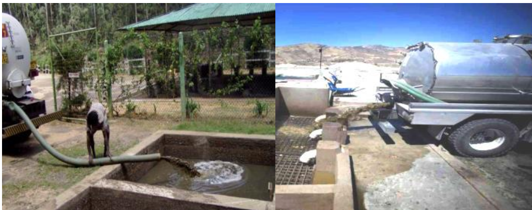
Figure 13 Sludge disposal into inlet chamber of STP
