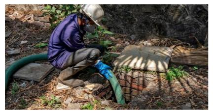
Figure 8 Desludger checking 25mm sludge depth is left in the septic tank after desludging
