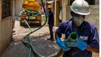
Figure 6 If the distance from the vacuum truck to the septic tank is long, two or three pipes are
