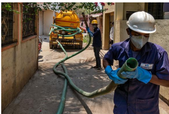
Figure 3- Desludging operations in Wai
