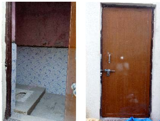
Photograph 3: Individual toilets constructed under SBM
