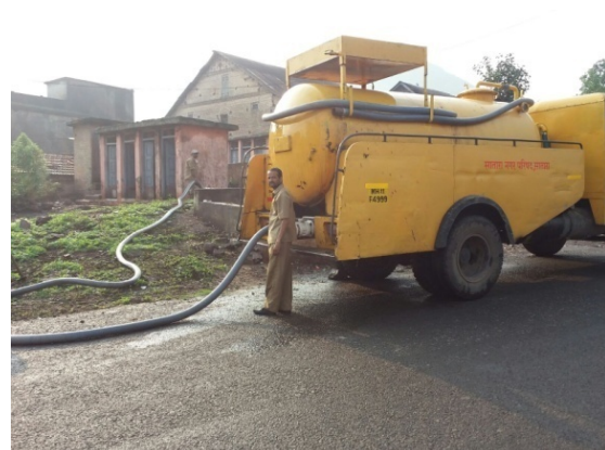
Photograph 7: Vacuum emptier for septic tank cleaning
