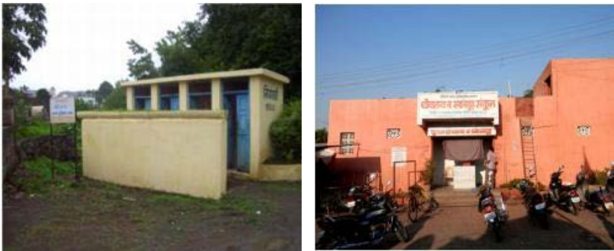
Photograph 8: Community toilets in Satara
