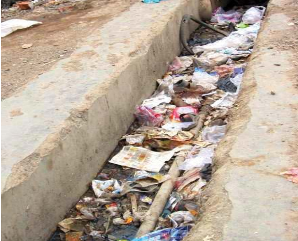
A side residual lane doubling as an open sewer
