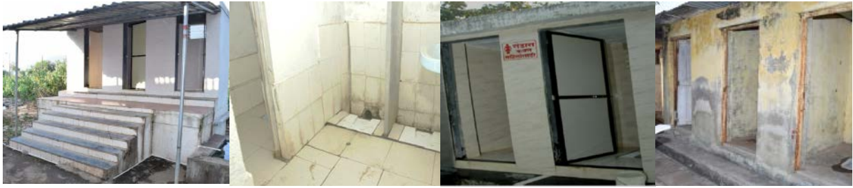
Photograph 8: Community toilets in Roha
