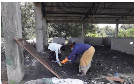
Dried sludge is further sieved for better quality compost
