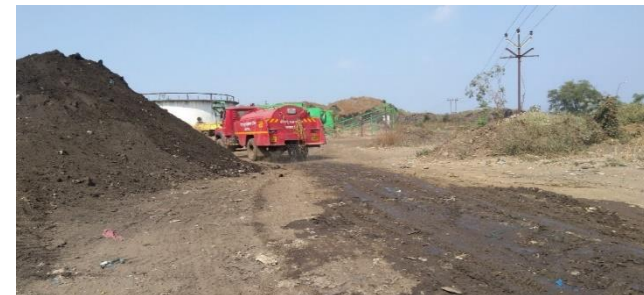
Figure: Reuse of treated wastewater from Kasaba Bawada STP to reduce dust problem at site
