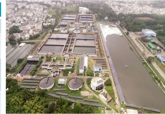
Figure: 245 MLD STP at Kabitkhedi
