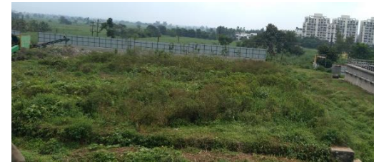
Figure: Sludge Drying Beds (not in use)
