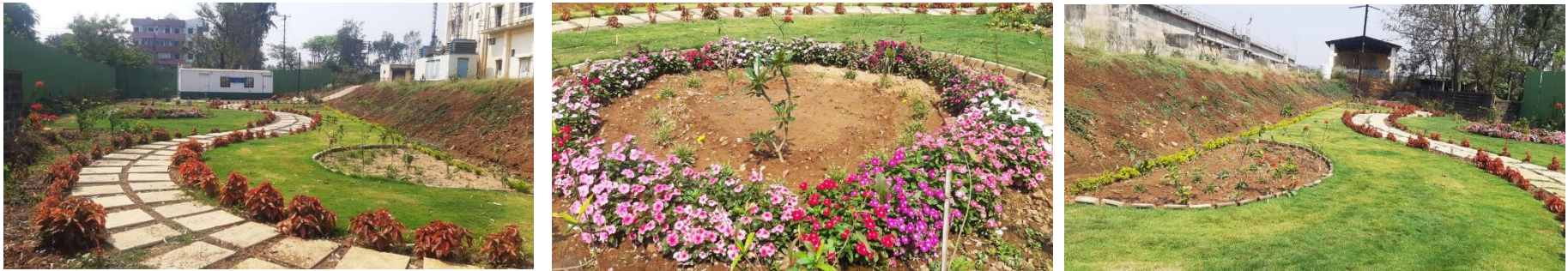
Figure: Reuse of treated waste water for watering of landscape at Kasba Bawda STP
