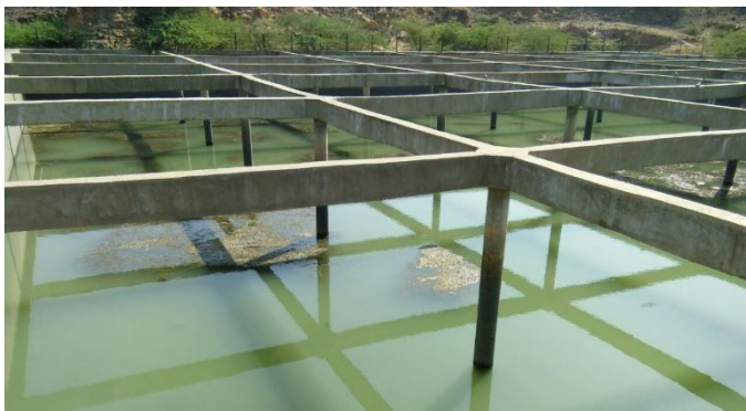
Figure 22: Narmada water storage tank at Kukma
