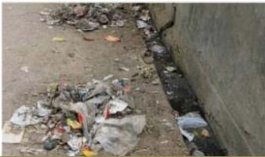
Clogged open drains
