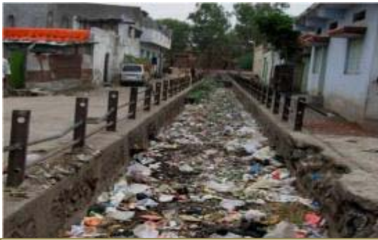
Clogged open drains
