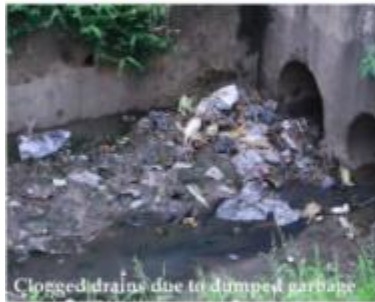
Clogged drains due to dumped garbage
