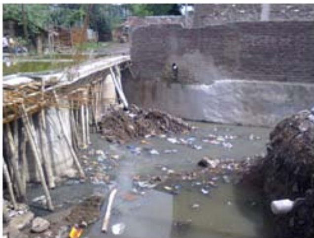
Photo Plate 3 Sanitation and sewerage in Beed
