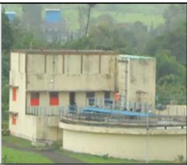
WTP at Chikhloli
