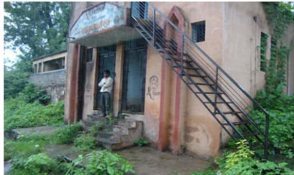
Community toilet in Achalpur
