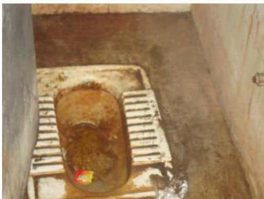
Community toilet in Achalpur
