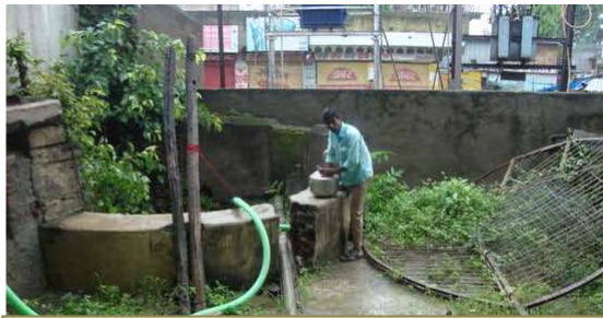
Water treatment at AMC
