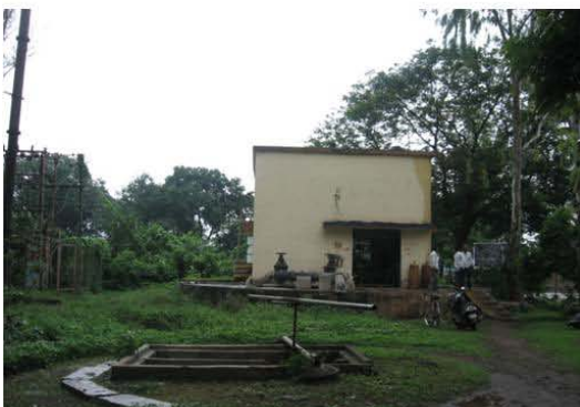
Water supply pumping station
