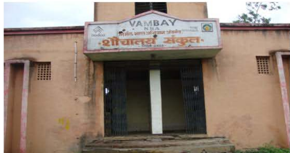
Community toilet in Achalpur
