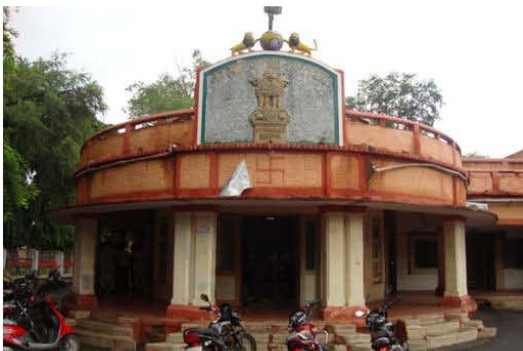
Achalpur Municipal Council Office
