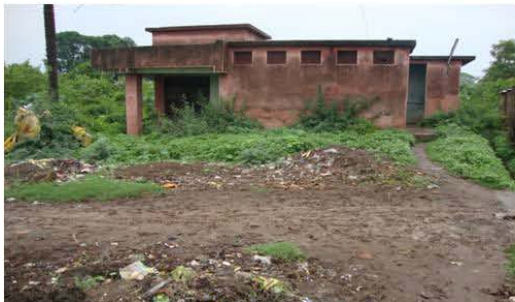
Community toilet in Achalpur
