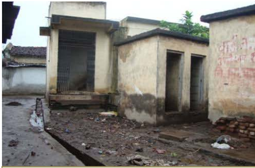
Community toilet in Achalpur
