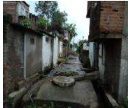
Septic tanks constructed on roads
