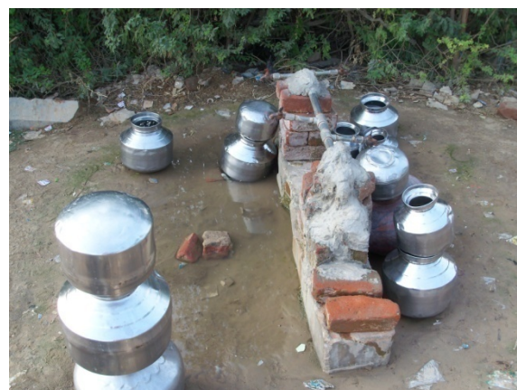
Figure 6: Community Standposts in Patan
