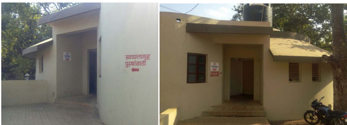
Image 4: Public toilet blocks in Panhala
