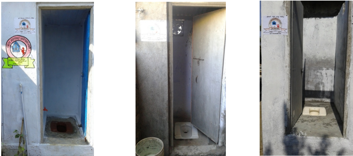
Photograph 3: IHHL Constructed under SMMUA
