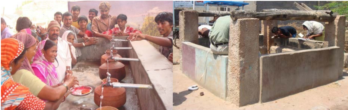
Photograph 17: Shivra Mandap public taps (left), Revitalized well (right)
