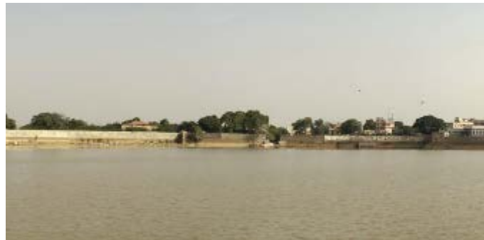
Figure 28: Repaired Hamirsar body wall
