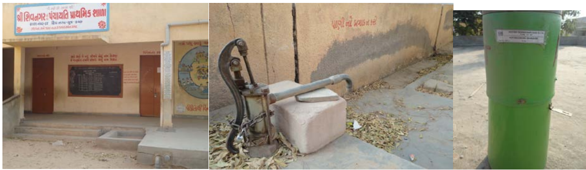
Photograph 18: Water tanks and handpump installed as part of RRWH at Shiv Nagar school
