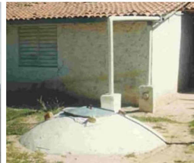
Underground lime and bricks cistern
