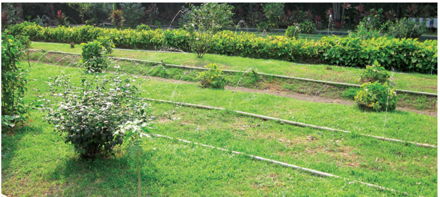
Trickling of wastewater through u-PVC pipes on the bioreactor
