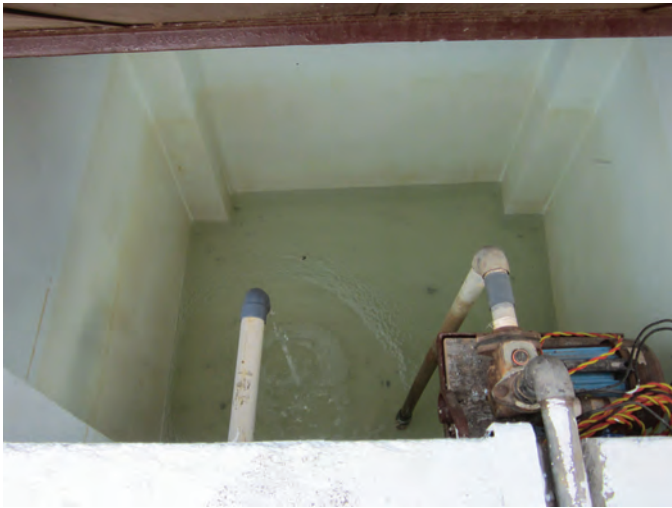
Collection tank of treated wastewater
