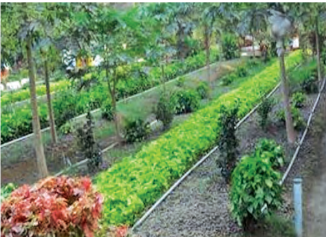
SBT based bioreactor for wastewater treatment at Naval Civilian Housing Colony
