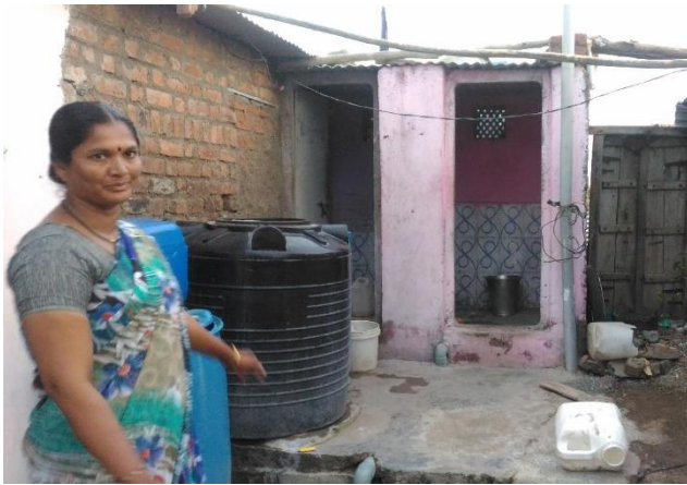
Archana has constructed a toilet and bathroom with plastering and tiling. Access cover for opening the septic tank is also properly placed. Cost of construction of the toilet was approx. Rs 50,000. She has borrowed Rs 11,000 from ICICI bank.
