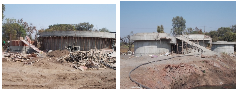
Photograph 10: Construction of sewage treatment plant, Malkapur
