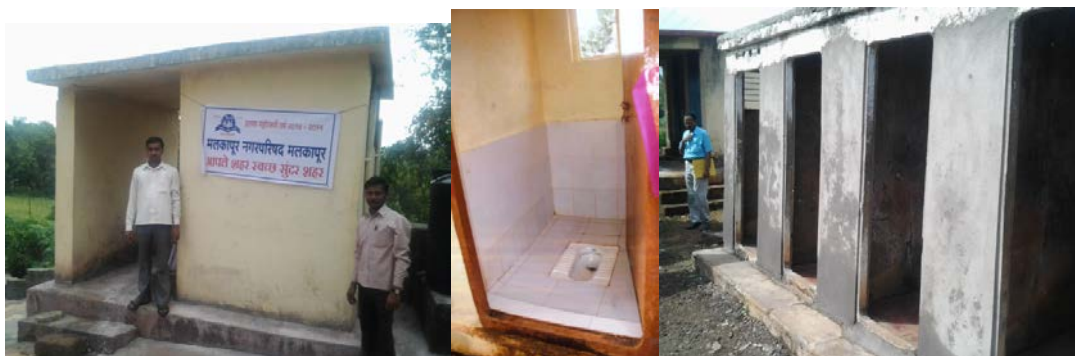
Photograph 1: Repaired and refurbished community toilets
