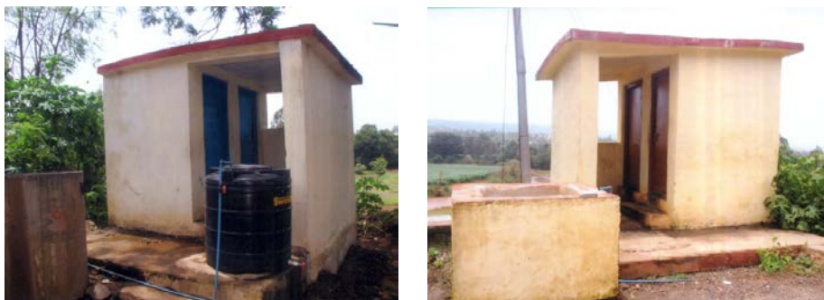
Photograph 5: Community toilets in Malkapur
