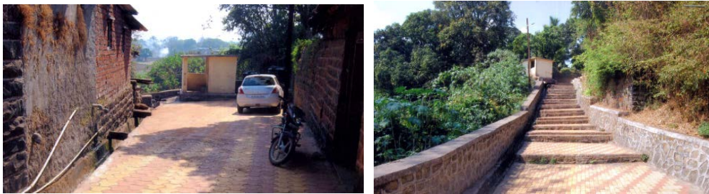
Photograph 7: Likely OD spots have been cleaned and paved to prevent OD
