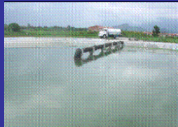
Sludge Lagoon System : 1 Nos
