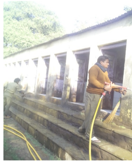
Photograph 2: Maintenance of CT
