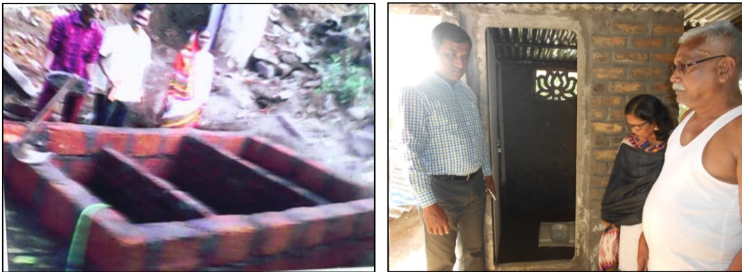
Photograph 6 and 7 - Water tanks constructed in community toilets
