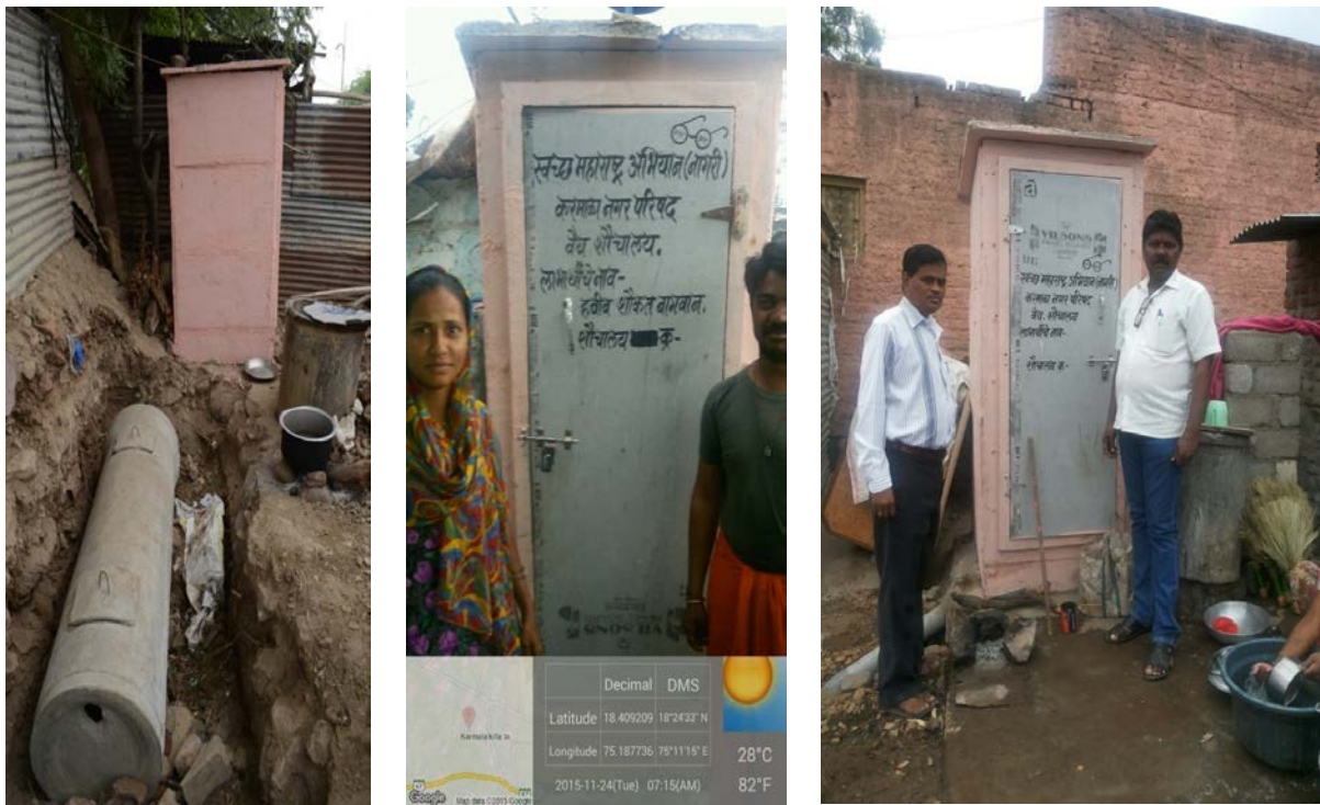
Photograph 4: Toilet construction under process and completion of toilet
