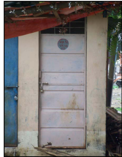
Figure 3: Locked community toilet in Borsad
