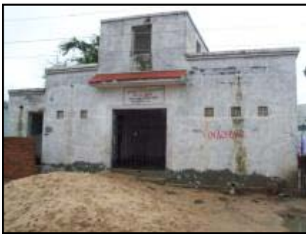
Locked community toilet in Harij
