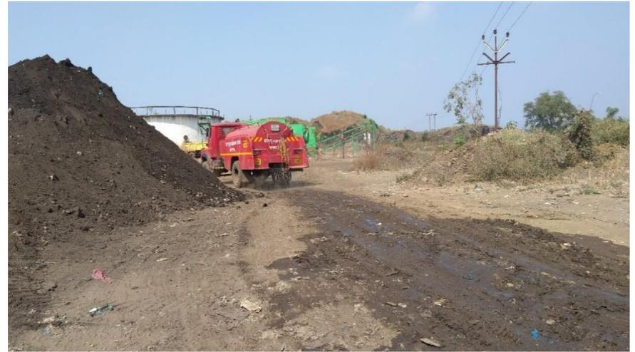
Figure: Reuse of treated wastewater from Kasaba Bawada STP to reduce dust problem at site
