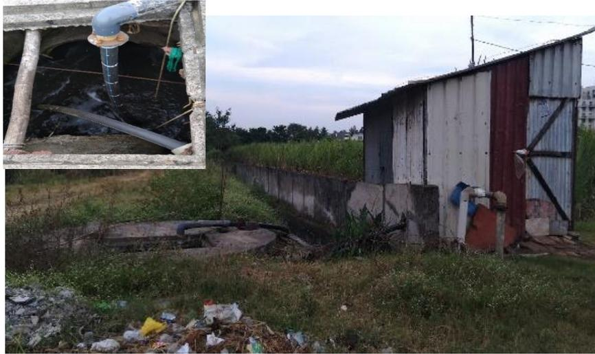
Figure: Pumping Station install by farmers to reuse treated wastewater from Kasaba Bawada STP through the chambers at treated wastewater drainage pipeline
