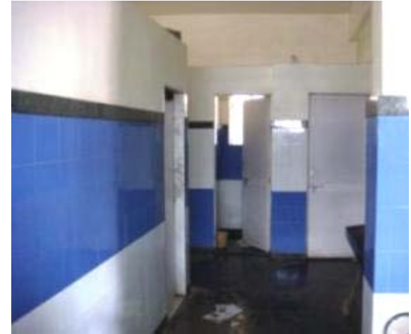
Clean pay and use toilets at Sinar Municipality bus stand premise
