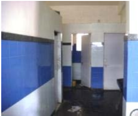
Contracting for management of community toilets
