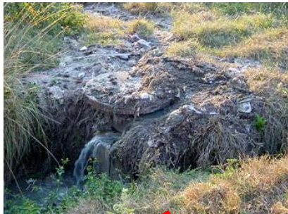
Overflowing sewer
