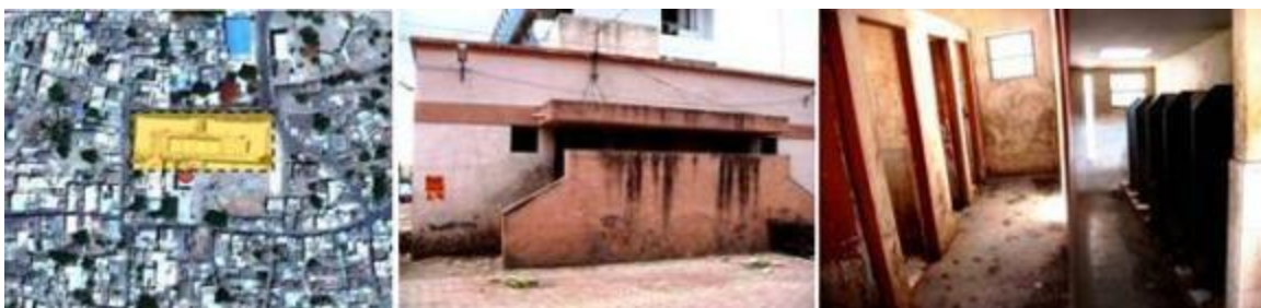
The public toilet in Market, near Nagar Parishad office.
