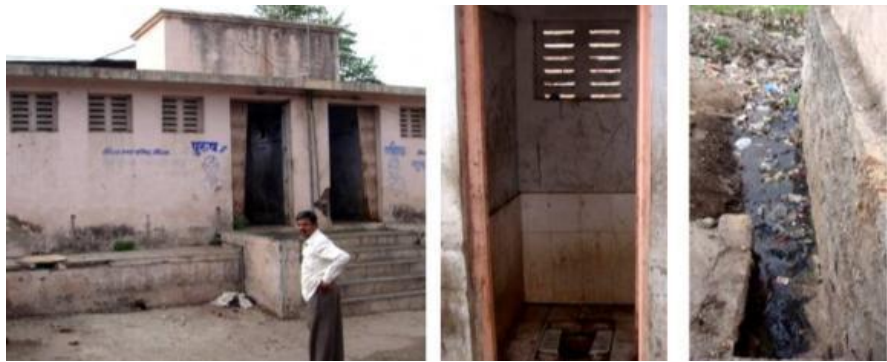
A public toilet block near Nehru Chowk in Sinnar.
