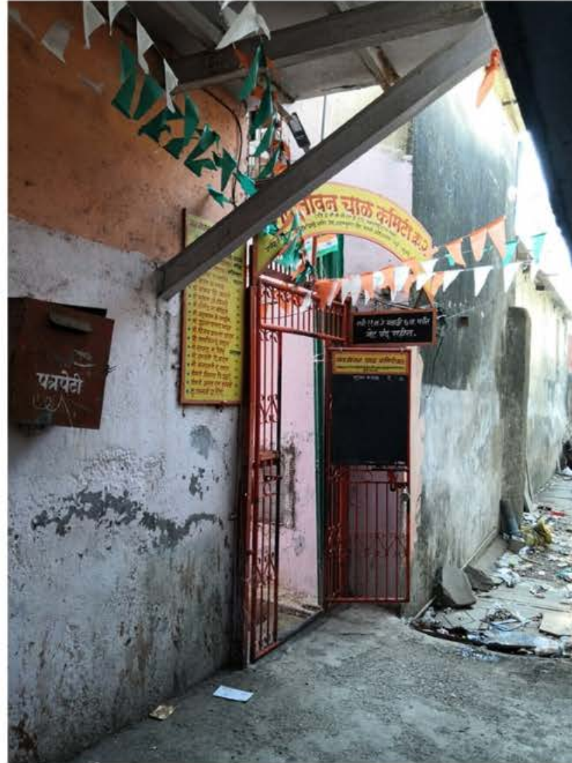
Forming gated societies to restrict the outsider from using the toilets
