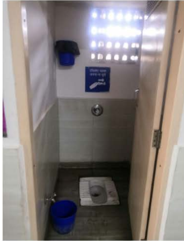
The clean and maintained toilet blocks with flush system, tap and dustbin available for each toilet seat
