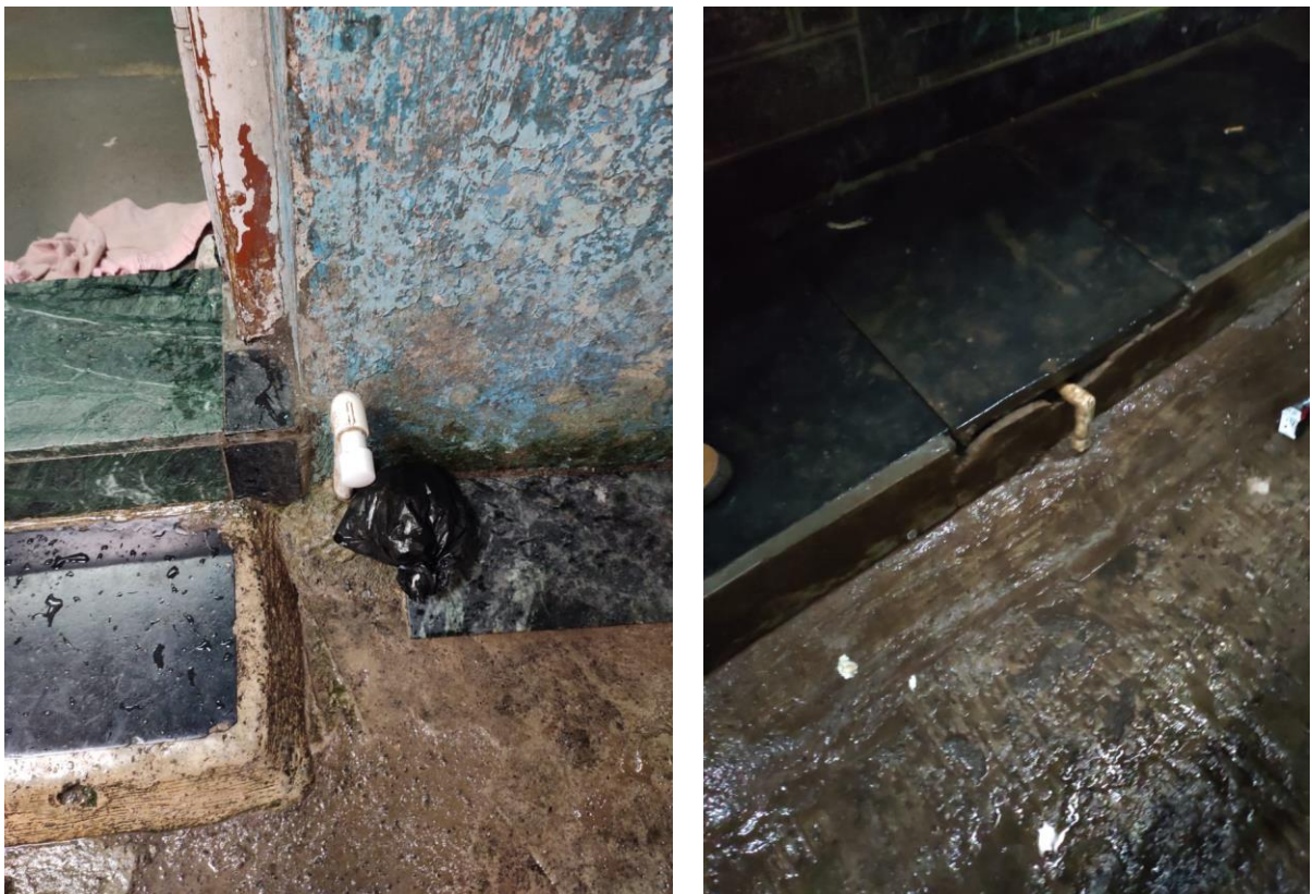
Figure 10 Water connection at household level in Dharavi and M-EAST slums
