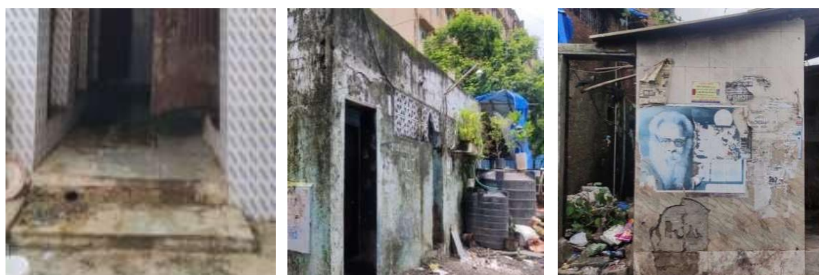
Figure 16 Bad condition of community toilets with no electricity
