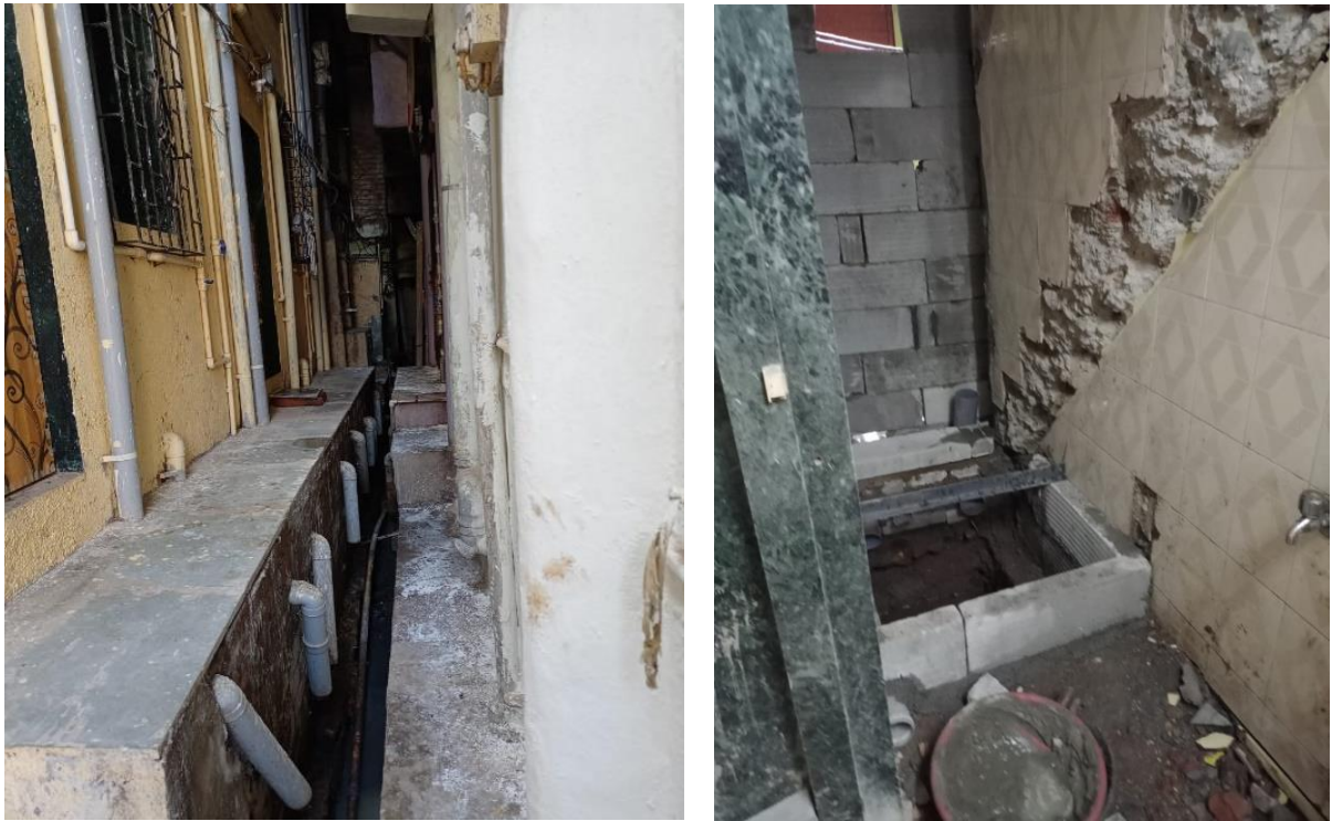
Figure 9 Waste from IHHT let into open drains & construction of IHHT in M-EAST slums
