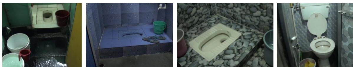
Figure 28 Individual toilets constructed by households
