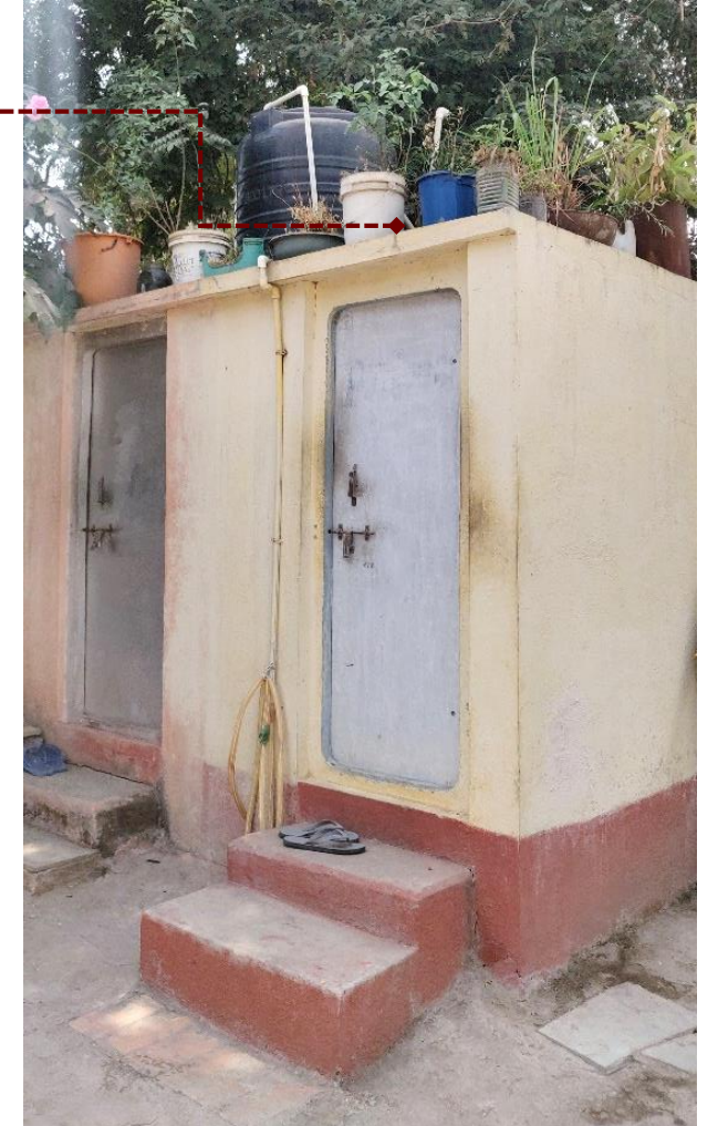
Household Toilet Built under SBM
