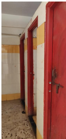
The toilet has working locks and doors, which makes it safe for the users.
