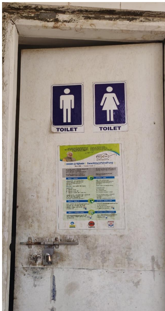
Petrol Pump Toilet
