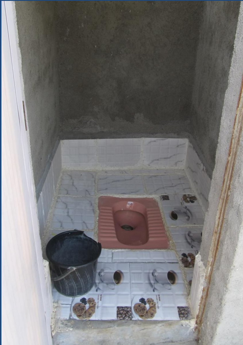
Inside condition of Toilet
