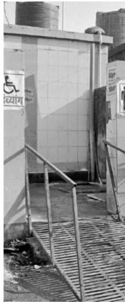
Public Toilets Probable requirement: 20000 L/ day
