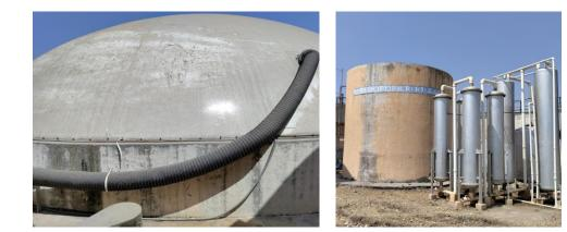
Methane generated from anerobic digestion is used for electricity generation (450 KW) and electricity is reused in the STP
