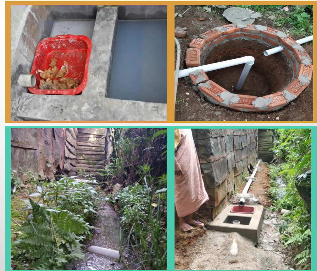
Before and after representative photograph with an adequate containment chamber after the user interface
