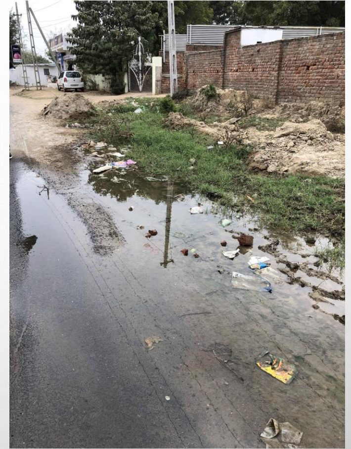
Spillover can be prevented by regular timed maintenance.
