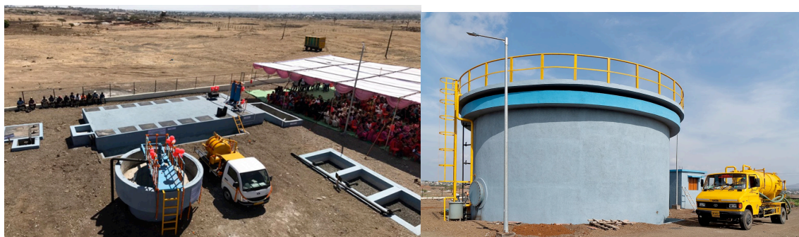
Figure 44: Treatment plant in Sinnar, Maharashtra
